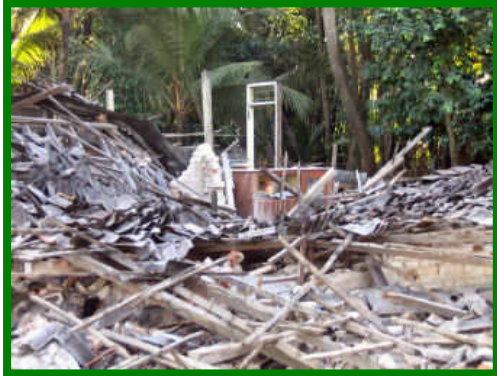
Yogyakarta Earthquake May 2006
